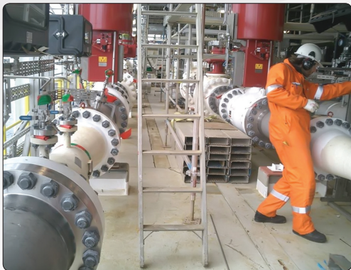
Installation of SPO CF spools onboard Sleipner R platform
